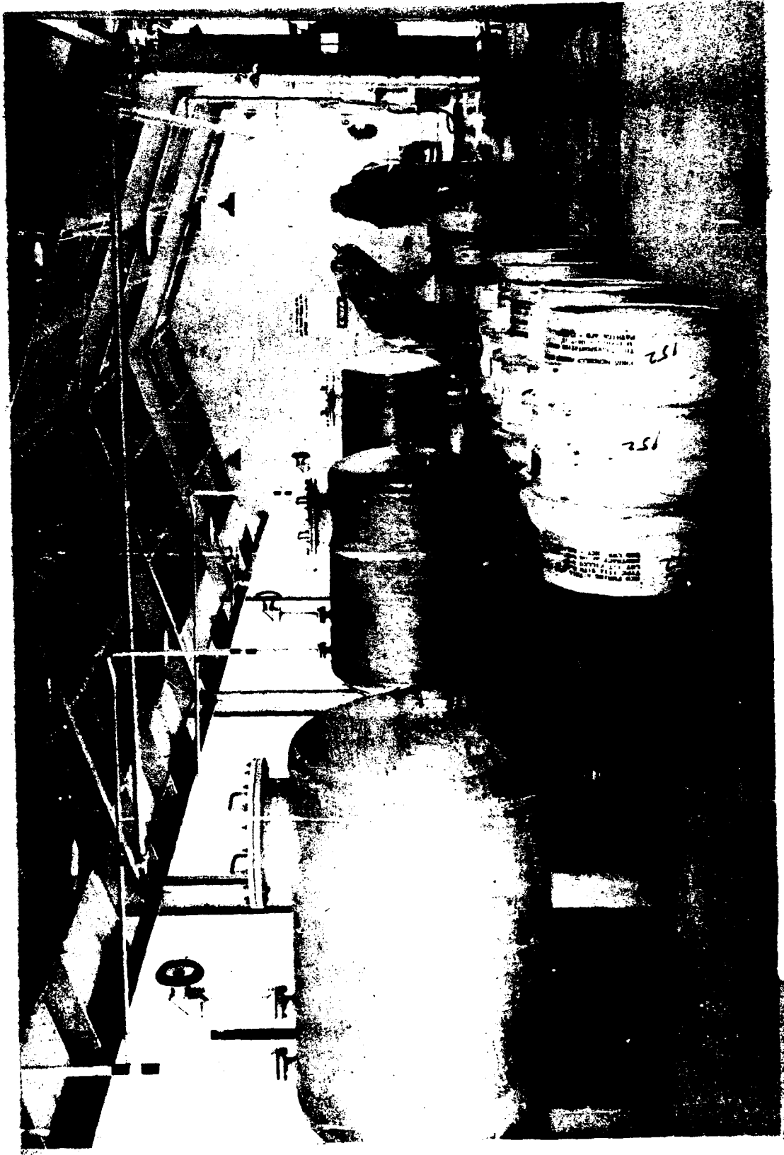
FIGURE 22 FUMING NITRIC ACID STORAGE TANKS AND DRUMS
