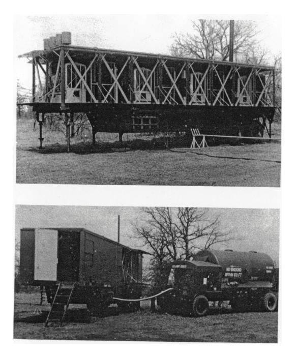
Figure 38. Liquid oxygen (LOX) is produced by the Redstone group's organic Engineer company. The generating plant consists of an air compressor unit (top photo) and an air separation unit (bottom photo) where the major components of atmospheric air, nitrogen and oxygen, are separated. The liquid oxygen is then routed to the liquid oxygen semitrailer (also shown at bottom) for delivery to the missile firing position.
