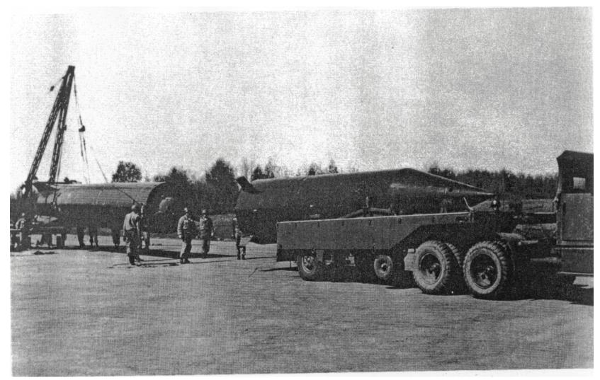
Figure 28. During missile assembly, the erector-servicer holds the missile thrust unit while the body unit is properly positioned by maneuvering the body unit (warhead and aft unit) trailer.
